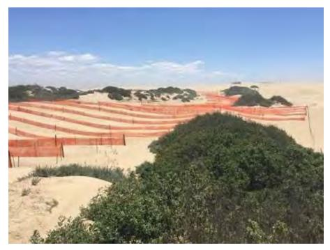
Photograph 12: Dust control program wind fencing at Tabletop
